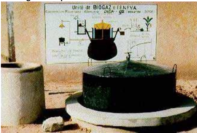
Figure 7: Floating-drum plant in Mauretania
